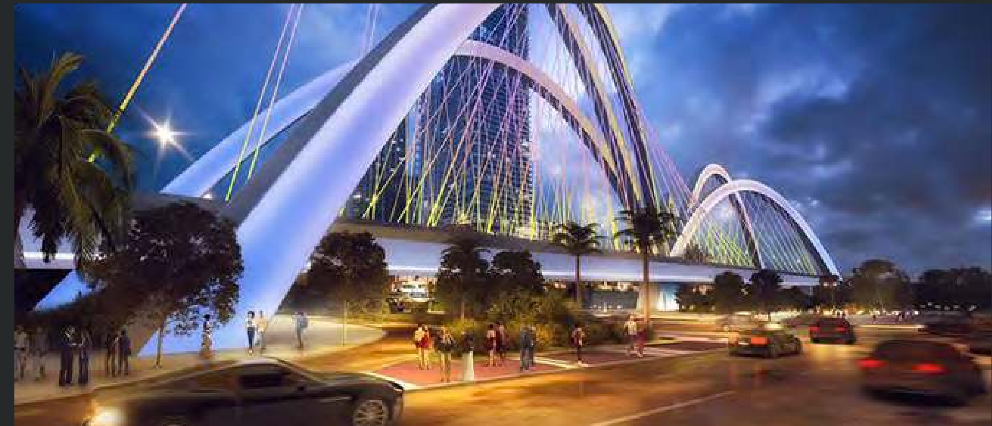
I-395 SIGNATURE BRIDGE
